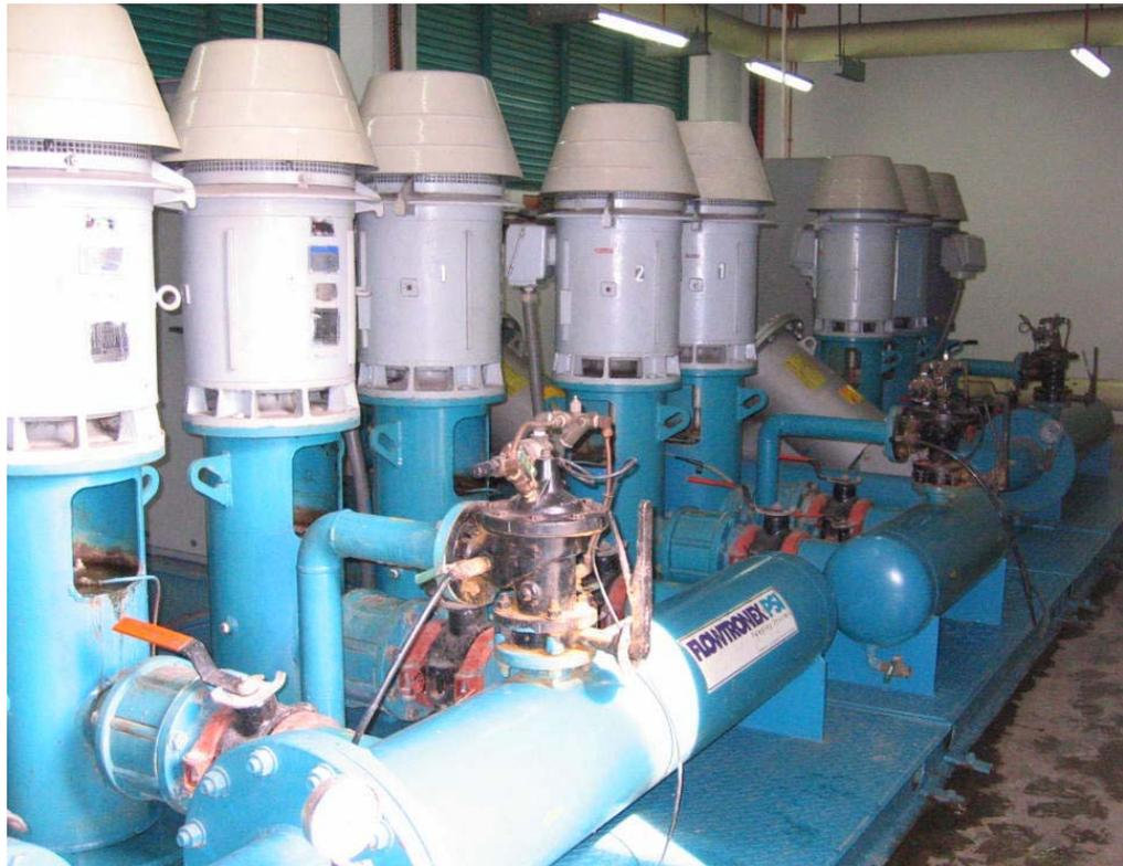
*The (3) Irrigation Pump Stations at the Singapore Turf Club (Kranji). The Watering Window for the main track is a tight 2 hours. The system (designed by Hydrogold in 1997) included watering for 5 different tracks as well as the extensive landscape irrigation of street verges for the surrounding complex.*
